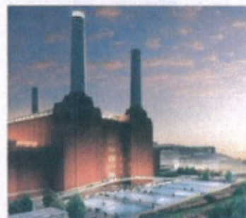
Focus On / The Power Station
